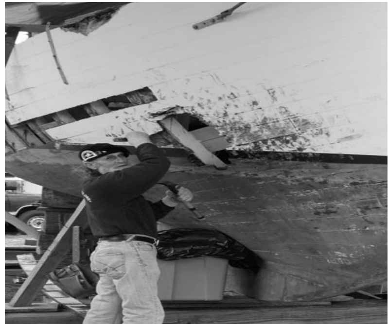
VFP56 member Jim Sorter removing damaged wood
